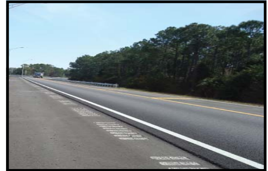
I-4 / I-95 Interchange - Daytona Beach, FL
